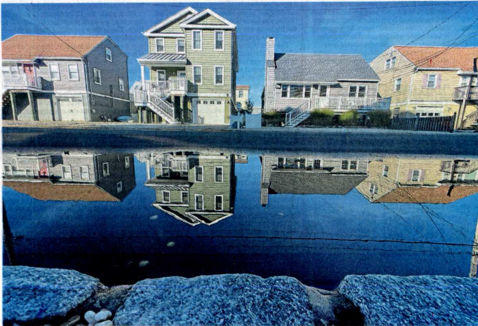
Long Beach Island houses — both rebuilt and elevated and old Cape Cods — on the unit block of West Sand Dune Lane on Oct. 6. The standing water is leftover from heavy rains in early October remnants of Hurricane Ian. Tom Gralish / Staff Photographer
