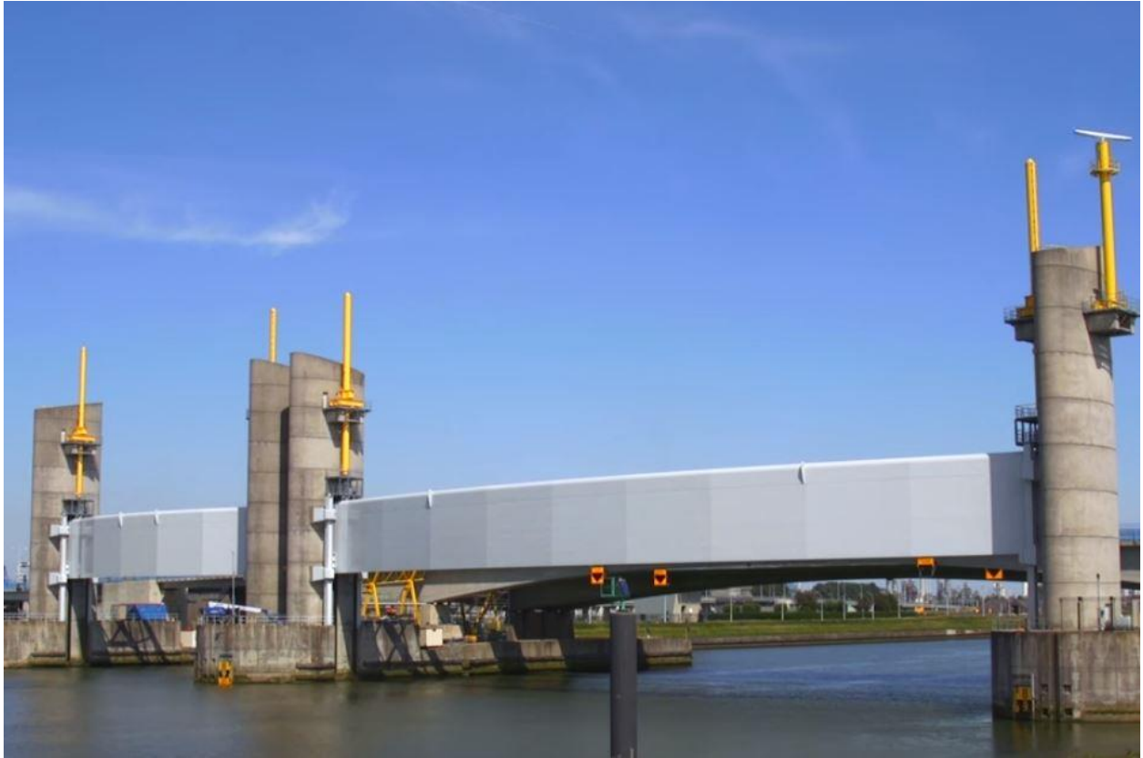
Figure 59: Hartel Barrier Vertical Lift Gates
